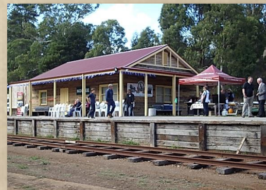
The reconstructed Noojee Railway Station and platform 2014
